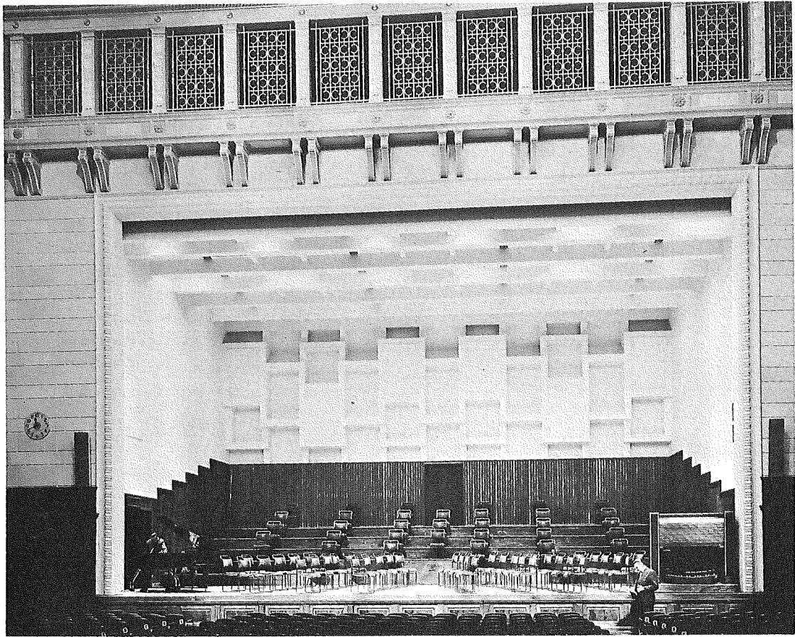
Fig. 6 - Stage of Southampton Guildhall after reconstruction, showing coffered walls and ceiling
